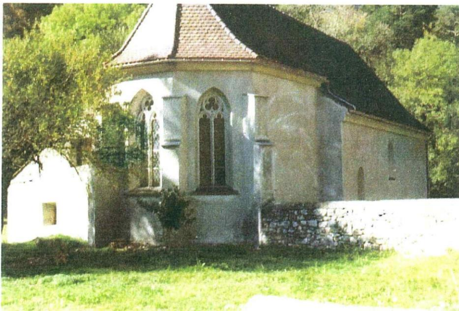
Rear of Community Church. 1977 photos.
